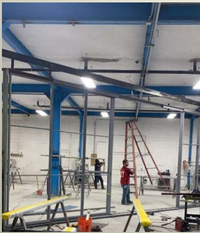
Door & Components Assembly/Inspection
